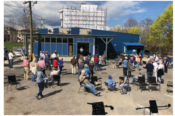
At a ribbon cutting event on April 19, 2021, members celebrated the completion of the Reuse Center building renovation.
